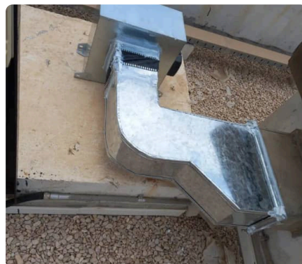
Galvanized ductwork
