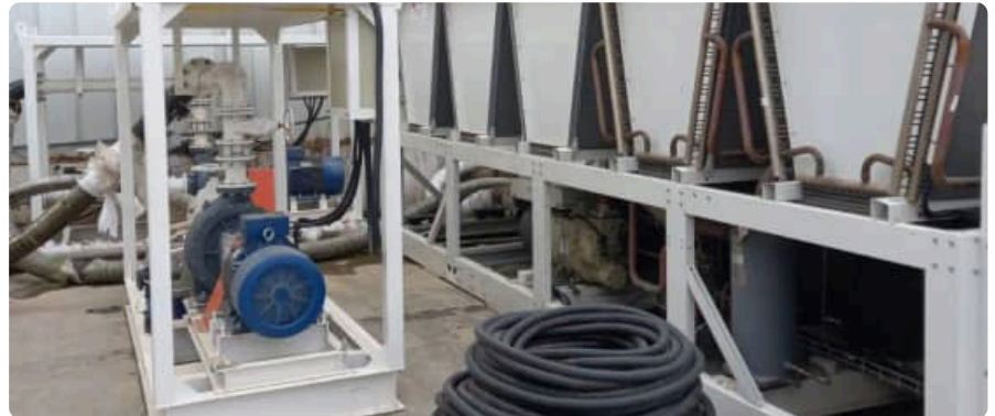
Chiller plant installation
