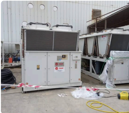
New chillers being installed
